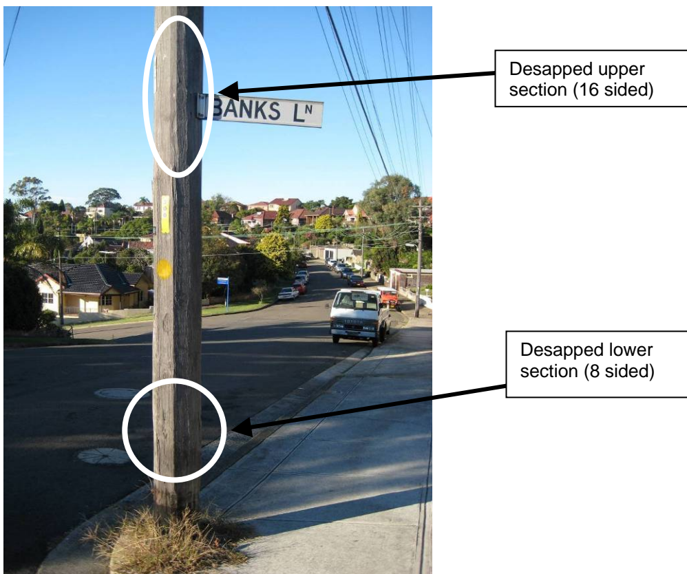
Figure 2: Desapped power pole - Sydney
