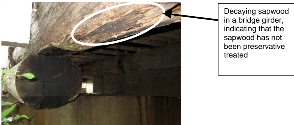
Figure 1: Sapwood which had not been preservative treated, decaying after a few years in service
